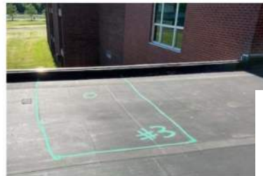
HS, Wet Area #3 (66 Sq. Ft.) with puncture circled within wet area.
